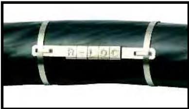
Marker Tags Installed on Power Cable
